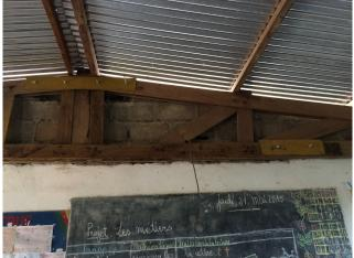
The new roof is at no risk of collapsing because the old wood is repaired and has been reinforced with brand new materials.
